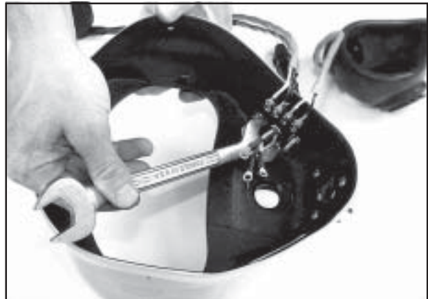
Fig. 6.19 Tighten the nut on the packing gland.
